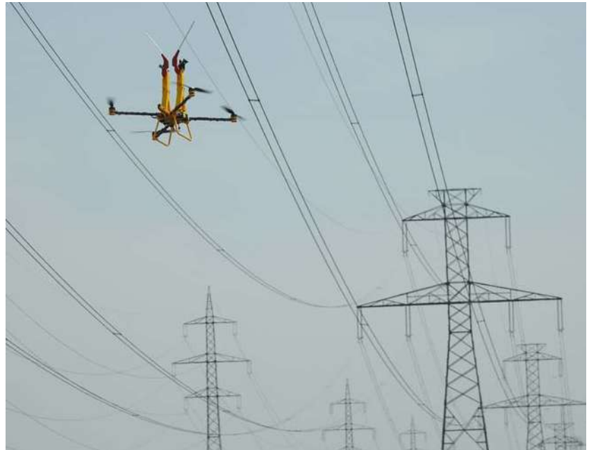
Image 7: Installation of the flight diverters on power lines with drone
