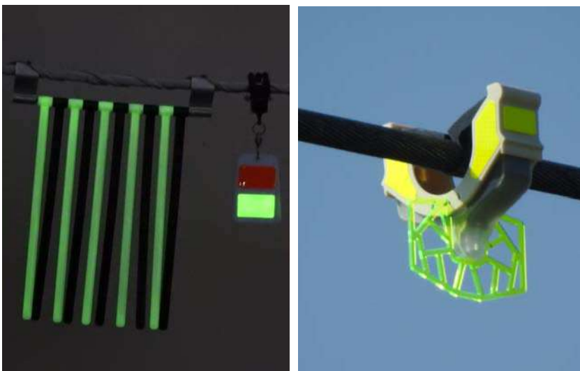
Image 6: RIBE lamella, FireFly and LED Diverter used to protect birds from collisions
