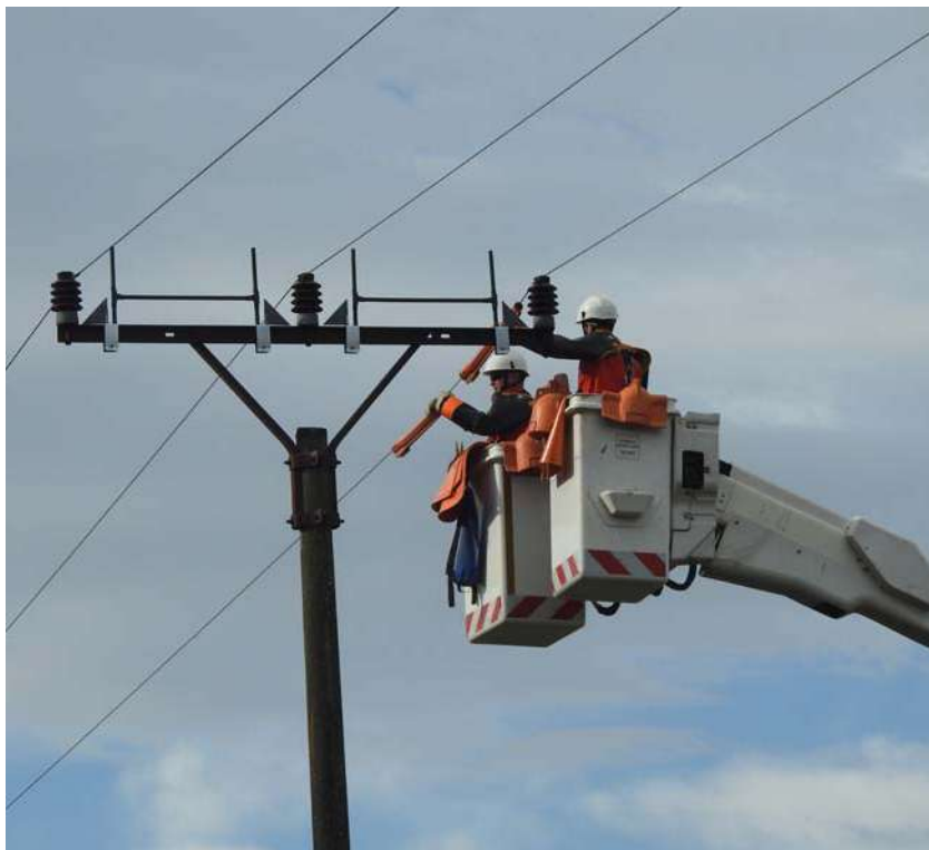
Image 9: Measures against bird electrocution – covering conductors with insulation materials and installation of rigid plastic covers for safe perching of birds
