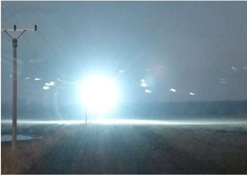
Image 5: Collision of swan into power lines often causes outages
