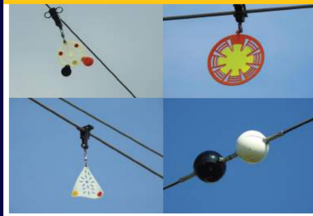
Several types of bird flight diverters were used, new types were developed and tested.
