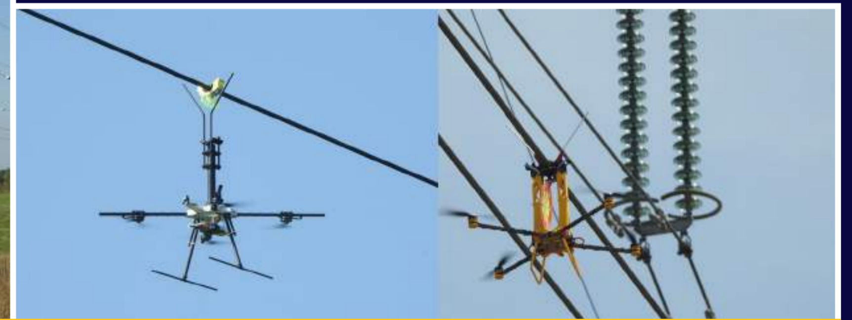
Different methods of installation of bird flight diverters were applied.
