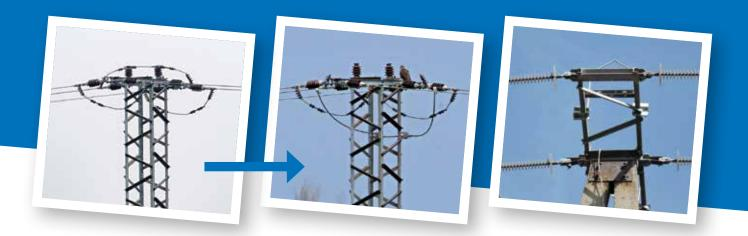
Even the riskiest poles can be made more safe by only changing one exposed jumper wire for the suspended type. It is a simple, effective, and cheap solution applied on 22 kV poles in Slovakia. Bare wires are replaced with insulated ones, the mortality rate has been reduced to zero. Also in case of changing the insulator to the 800mm long new type, and using insulated power connections, the mortality could be eliminated from the most dangerous type, the tension poles.
